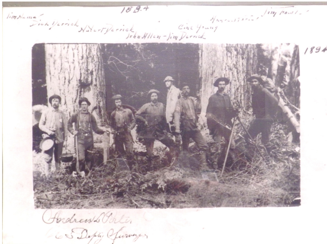
Field Crew of Contract 630 of Andrew L. Porter, T8S R8W, 1894. From Left: Jime Hume, Dick Derrick, Hubert Derrick, John Allen, Cine Young, Jim Derrick, Andrew Porter and Jim Fowler. Based on the scribing on the post, it appears they are at a closing corner and chopped a face that penetrated the bark of the tree on the BT. (Thanks to John Waffenschmidt, Lincoln County Surveyor)
